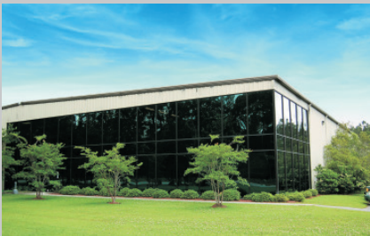
Plant III, Summerville, SC, USA
