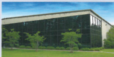
Plant III, Summerville, SC, USA
