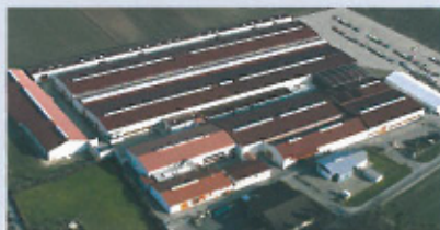
Plant I, Gremsdorf, Germany
