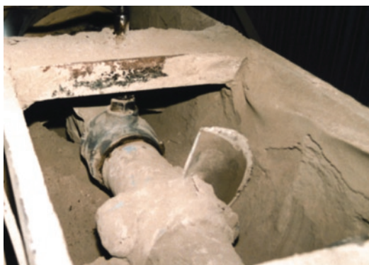
Hanger bearing on a gypsum scroll conveyor
