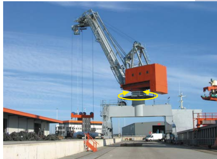
Harbour cranes, mobile harbour cranes
