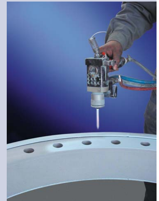
Metal zinc spraying (flame spraying) on sand-blasted surface
