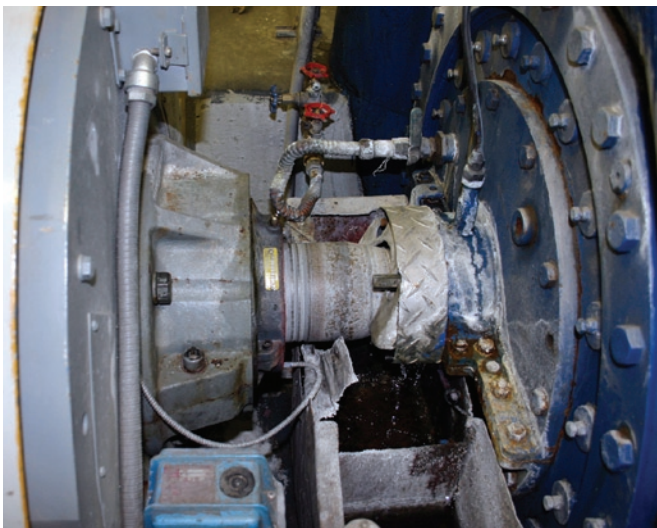
Cooper round flange in a trapped location
