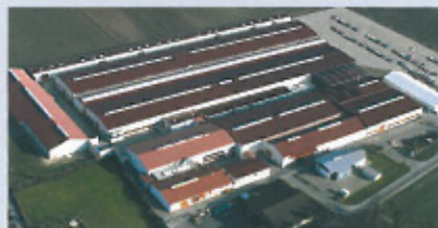
Plant I, Gremsdorf, Germany
