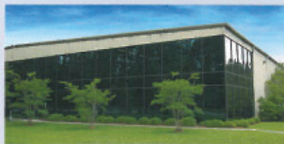
Plant III, Summerville, SC, USA
