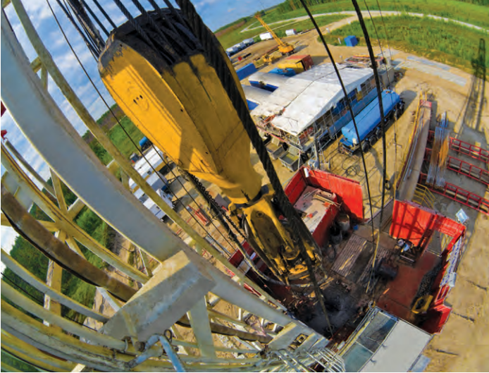
Rotating Rig Equipment
